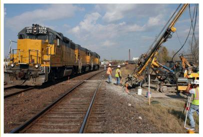
Graph 30. Jet grouting of piles/columns under an existing railway to compensate for very soft ground.  $\odot$  Hayward Baker, Inc., photographer: Jeffrey Hill.
