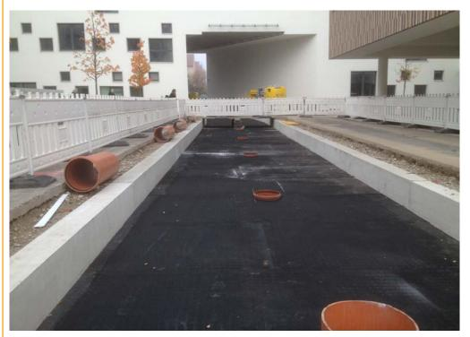
Graph 22. Example of an under-ballast mat in a trough, here for a light rail track in Munich, Germany (© Calenberg Ingenieure).
