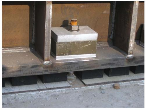
Graph 35. Example of elastic bearing in building foundation (source: CDM Group)
